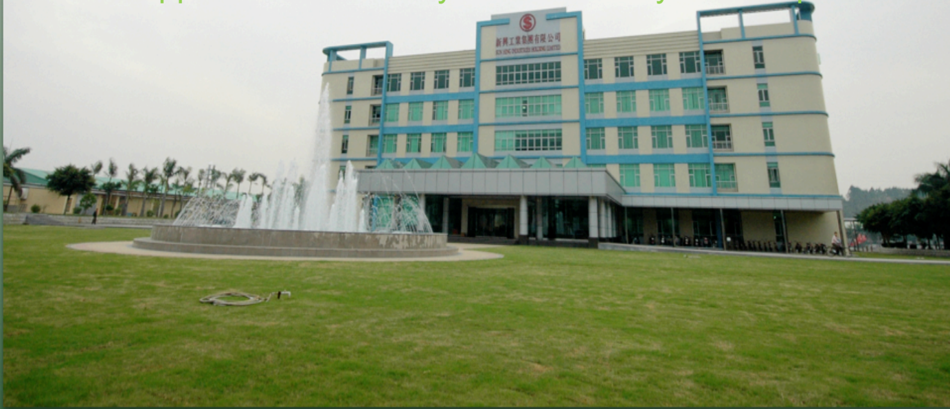
Underground anaerobic oxidation pond ( beneath the fountain )
